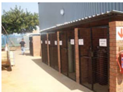
Brick building with four compartments with lockable gates for security
