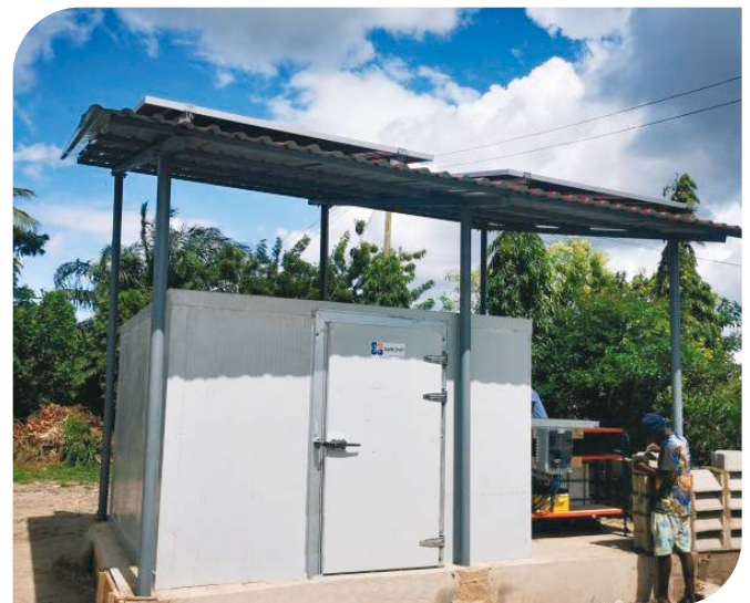
Figure 1 | SelfChill solar cold room in Tanzania. (© SelfChill)
